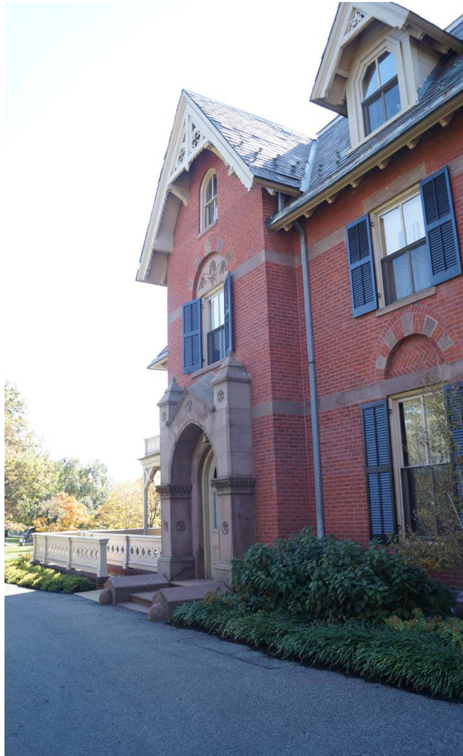
12. View of the front entrance into House 1
