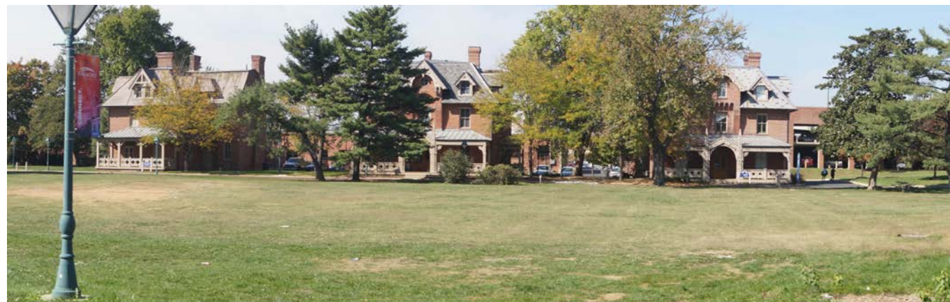
2. View of Parking Garage from the northern edge of the Faculty Row houses 3. View of Faculty Row houses from Olmsted Green
